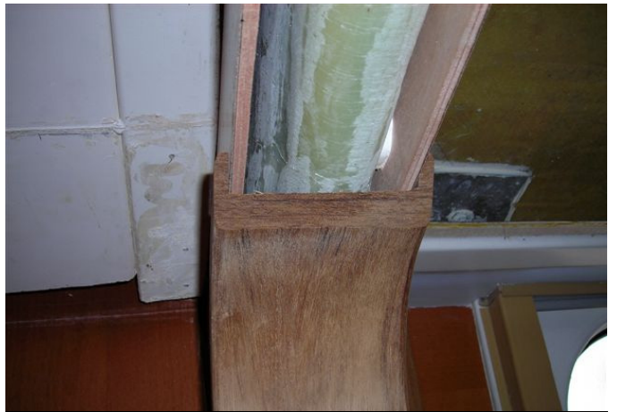
New bulkhead with trim temporarily fitted.
